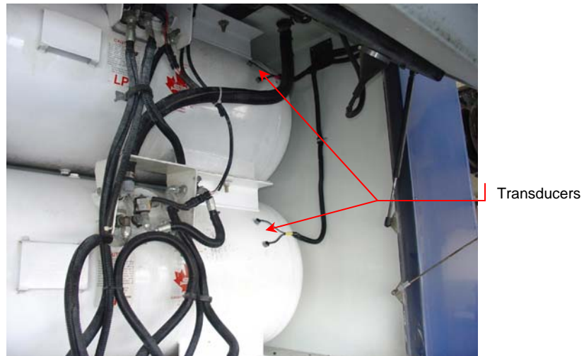
Fig. 7. Permanently Installed Transducer on Two Rear LP Gas Bus Tanks
